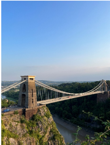
Clifton Suspension Bridge
